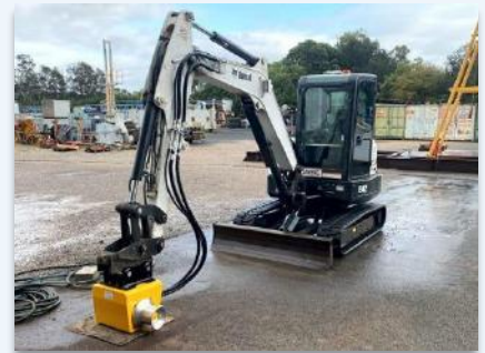
Quick-Hitch Capstan Winch Mounted on an Excavator
